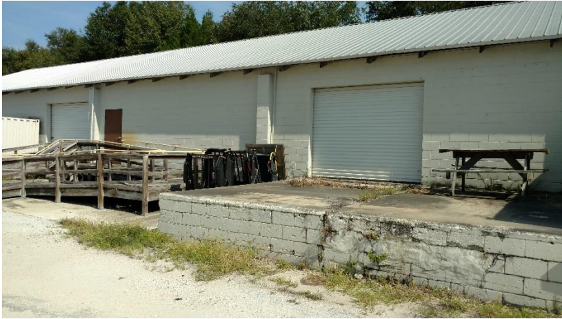
Large storage building located on Ride Solutions Inc. parcel.
