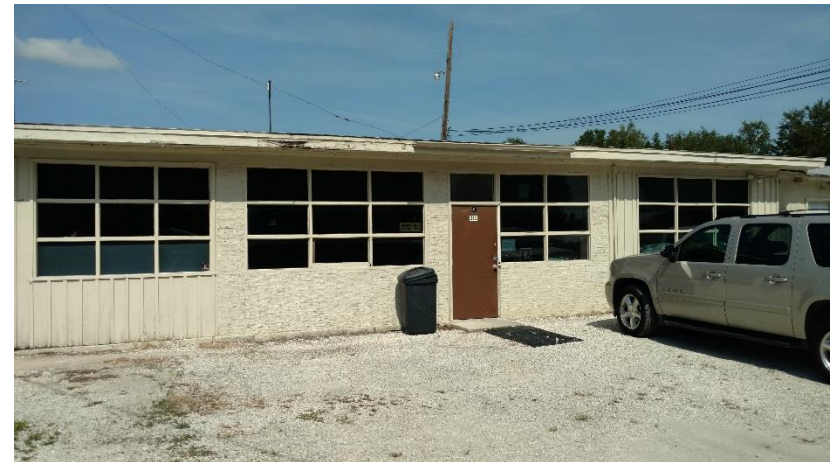
Former Ride Solutions Inc. offices now used as the drivers lounge area.
