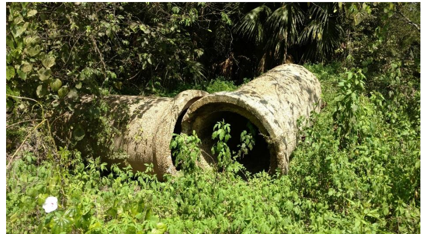
Discarded concrete pipes along road/path..
