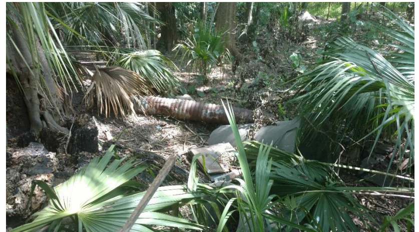
Corrugated pipe along berm in interior of parcel.
