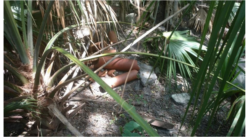
Clay pipe and concrete protruding through overgrown berm of soil and refuse and demo debris.
