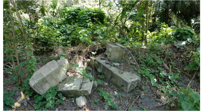
Demo debris mounded up in a berm on edge of road/path into the heart of the subject parcel..
