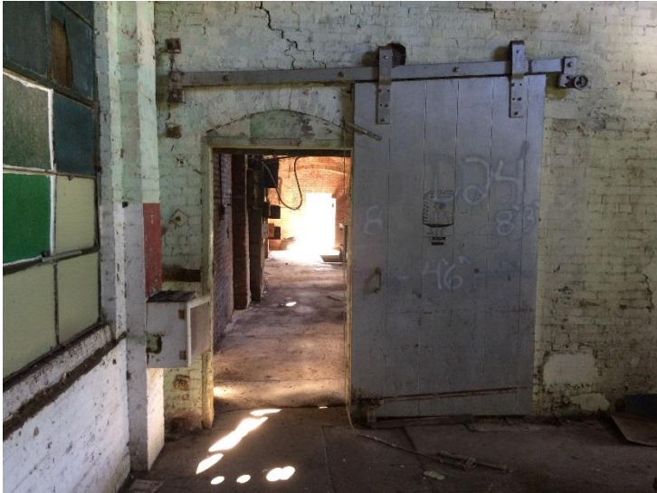
Looking into the boiler room.
