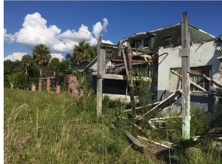
Back of main building.
