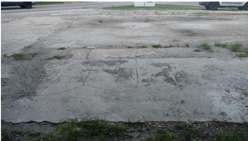
Former filling station floor and foundation footings
