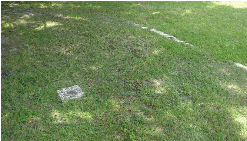
Former foundation footings and grass cover.
