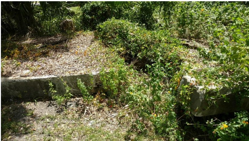
The footings and foundations of small building in south portion of property.
