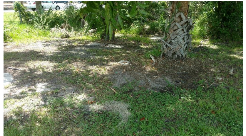
Several AST tank cradles now overgrown with trees and grassy vegetation.
