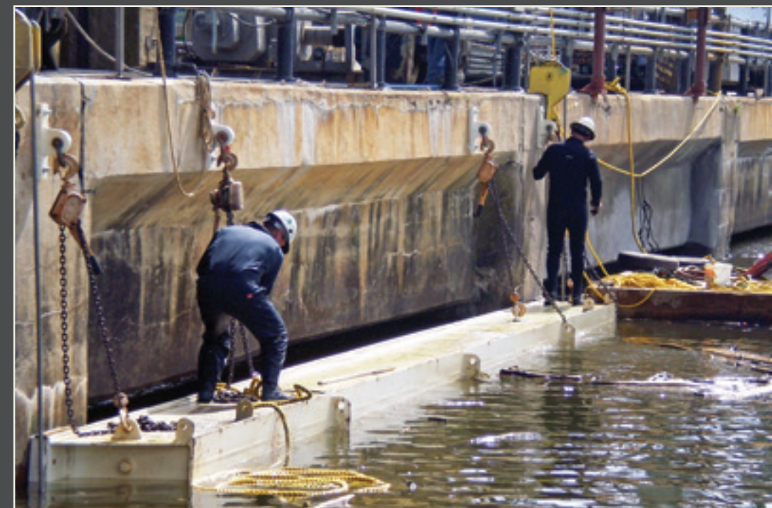
Crews at the Conowingo Dam move the bulkhead into position.
