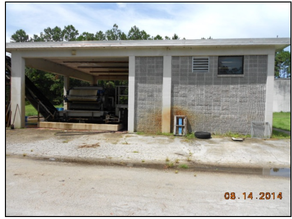
DEWATERING BLDG SOUTH
