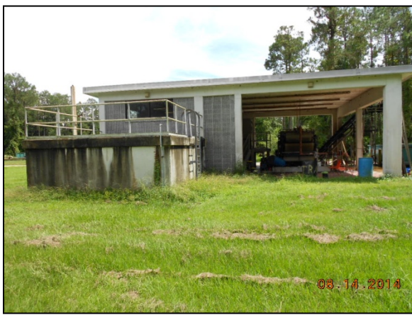
DEWATERING BLDG NORTH
