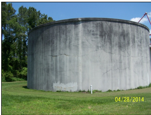
DIGESTER TANK (WEST) EXTERIOR
