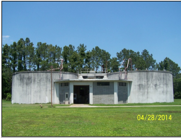
SLUDGE DIGESTERS / CONTROL BLDG
