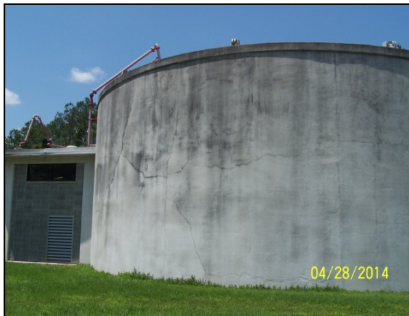
DIGESTER TANK (EAST) EXTERIOR
