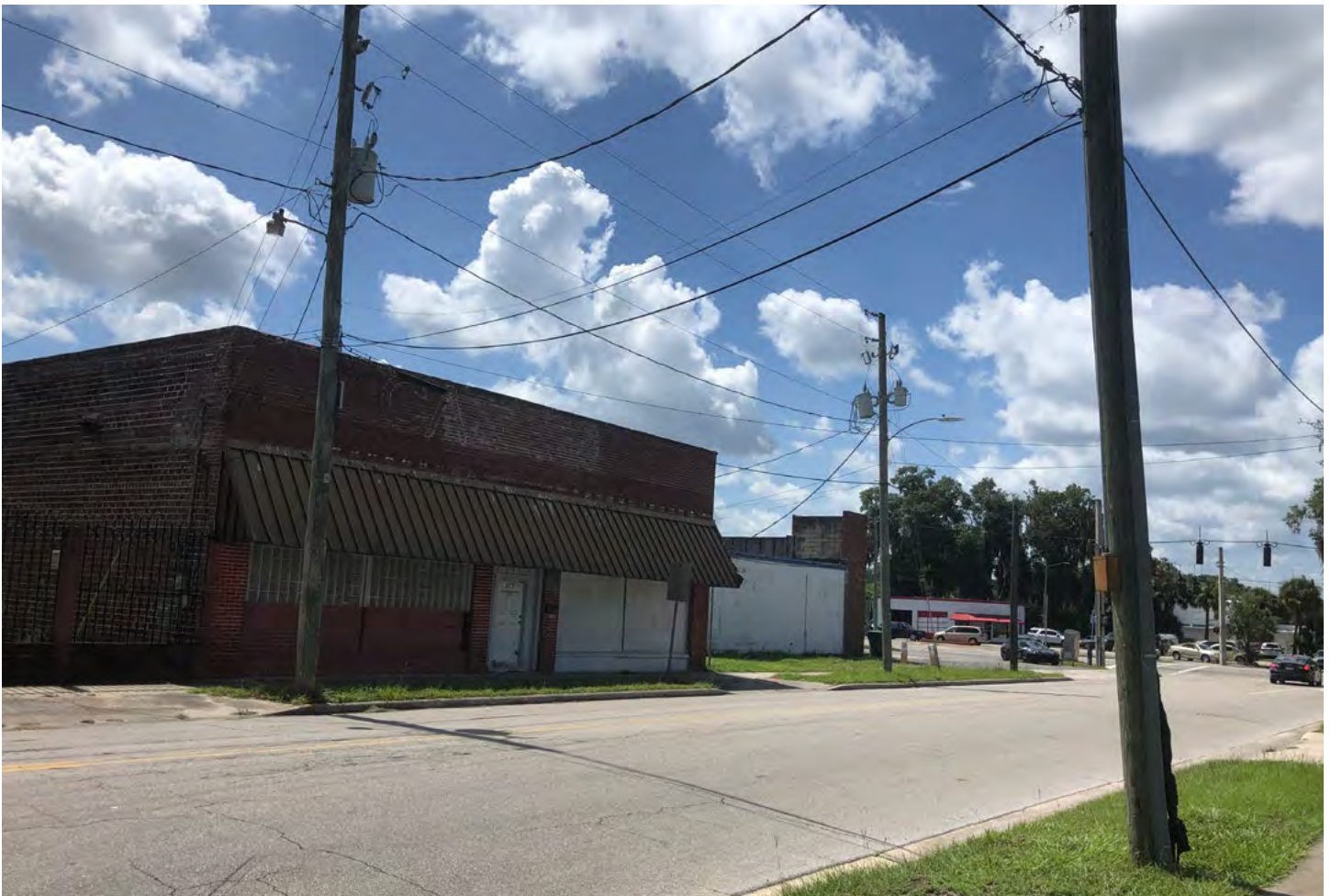
Image 9 Vacant Building in Palatka, FL
